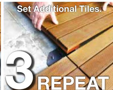
During installation, use the entire connector; use halves or quartered tile connectors on hidden and exposed edges including corners. Use the edge of the spacer to provide a gap between your new tiled deck and any adjacent structure such as a house, fence, or wall.
